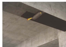
Carbon Fiber Installation
